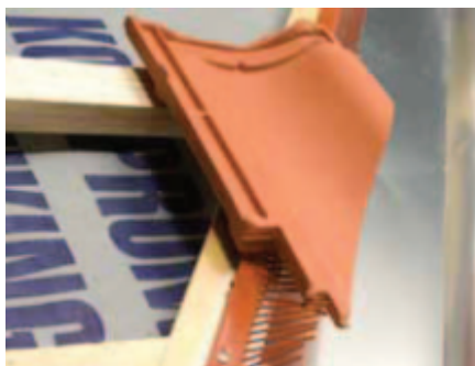
The Eaves filler comb is placed no more than 20 mm from the edge.
