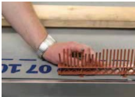
The Eaves filler comb is placed no more than 20 mm from the edge.
