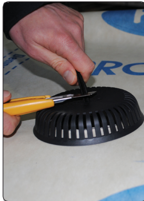
Cut the strip off approx. 1 cm above the grill.
