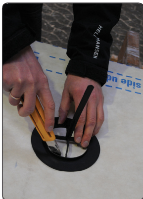
Mark and cut a hole in the underlay
