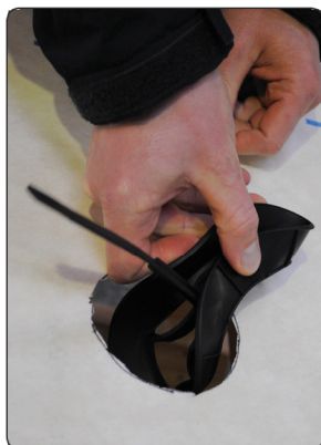
Squeeze the underpart of the kima-Air outside/in and push through the Hole, so that the underlay will be Between the under part (in) and the Grill (out)
