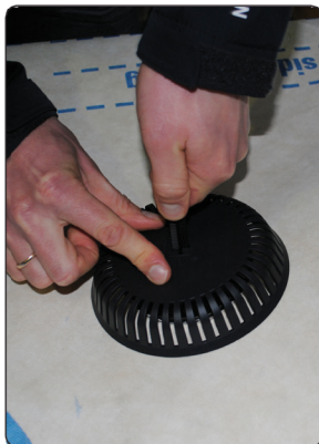
Press the grill against the underlay pull the strip to tighten
